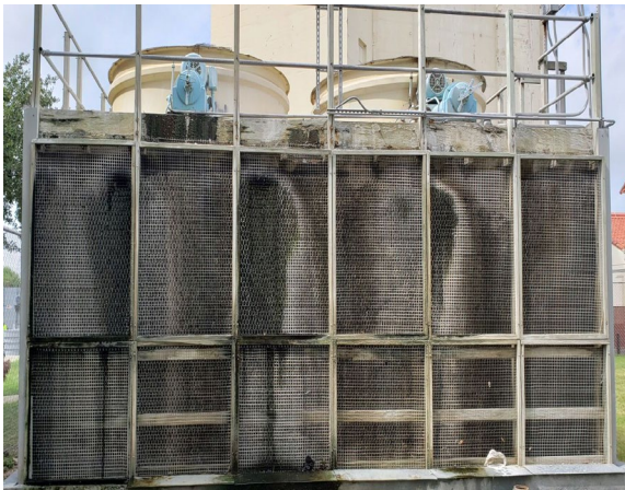
Cooling tower past its useful life
